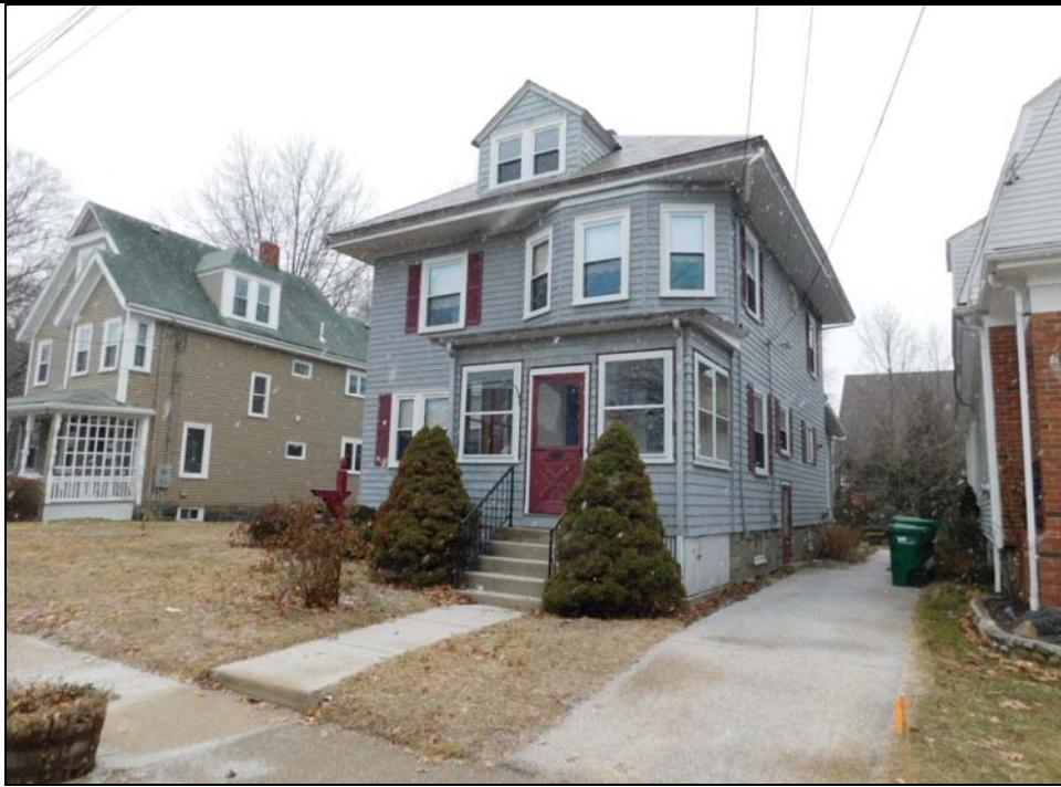
View from E showing N-facing elevation.
