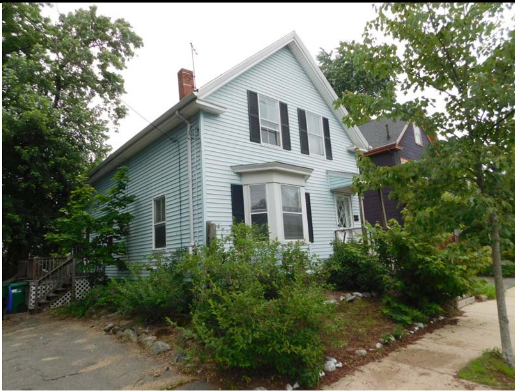
View from SW showing left elevation.
