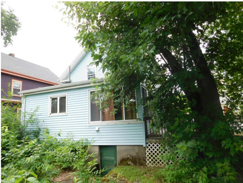
View from N showing rear elevation and ell.
