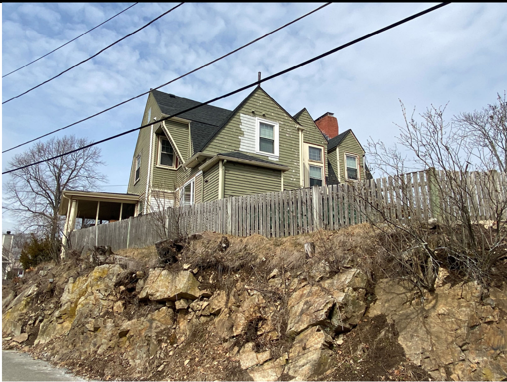
Rear elevation from the SE.
