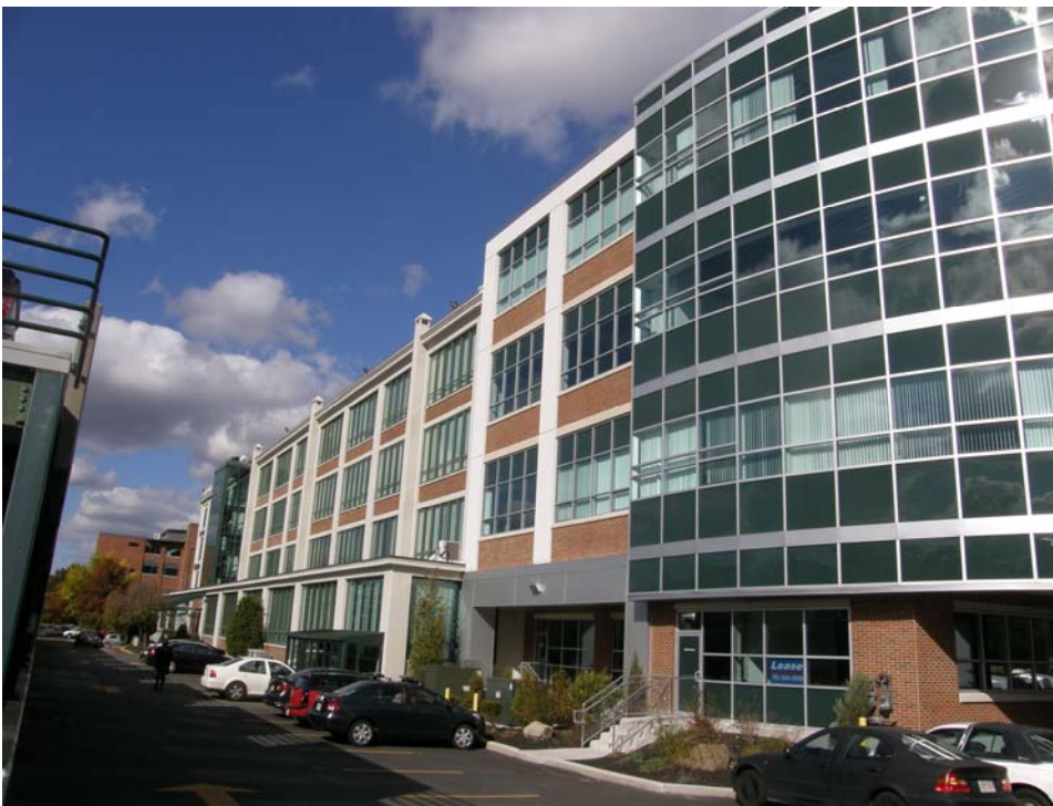
200 Boston Avenue, south elevation
