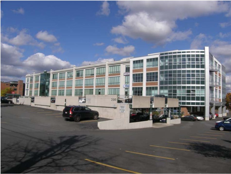
200 Boston Avenue, south elevation
