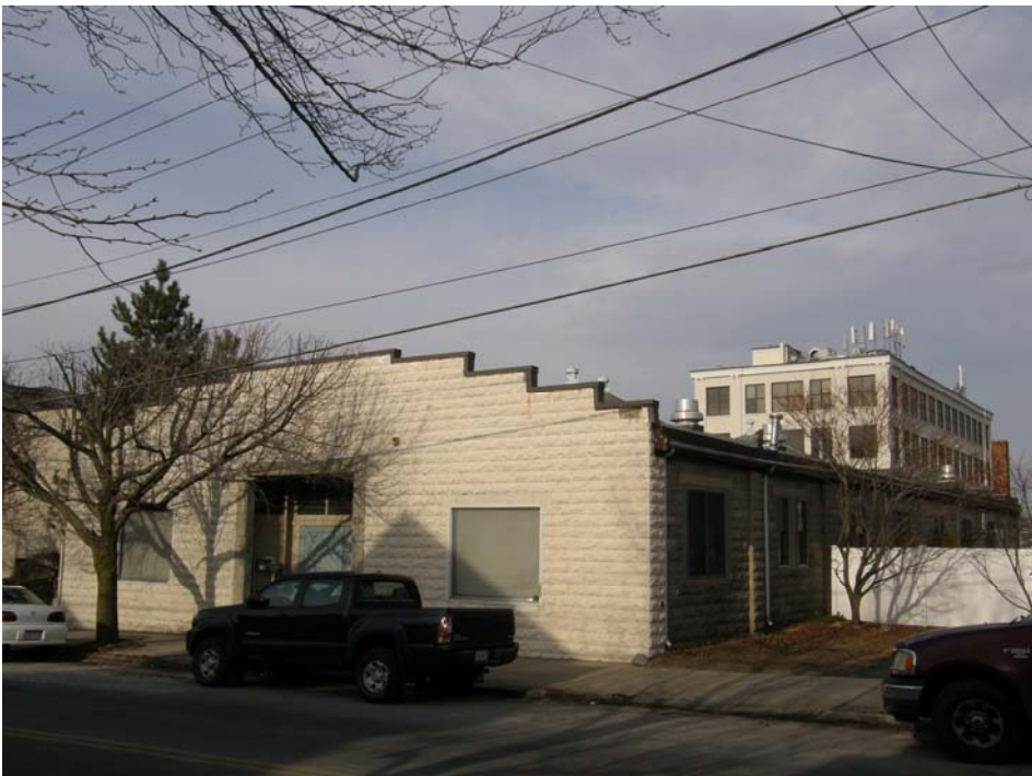
236 Boston Avenue, south elevation
