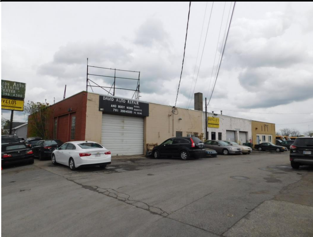
South-facing side elevation from S.
