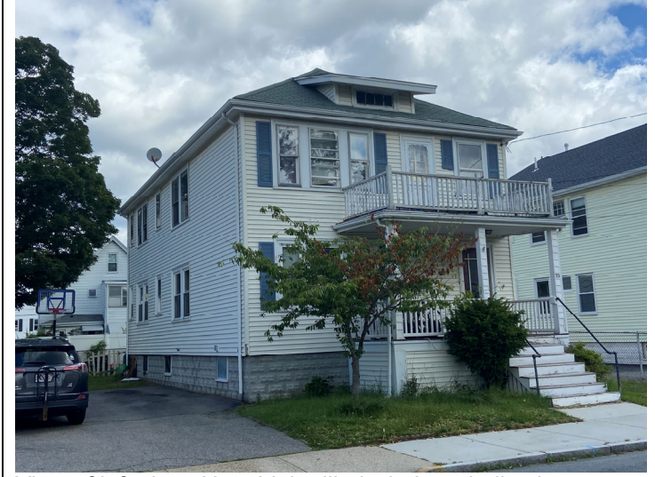
View of left elev. Note high-silled windows indicating a bath.
