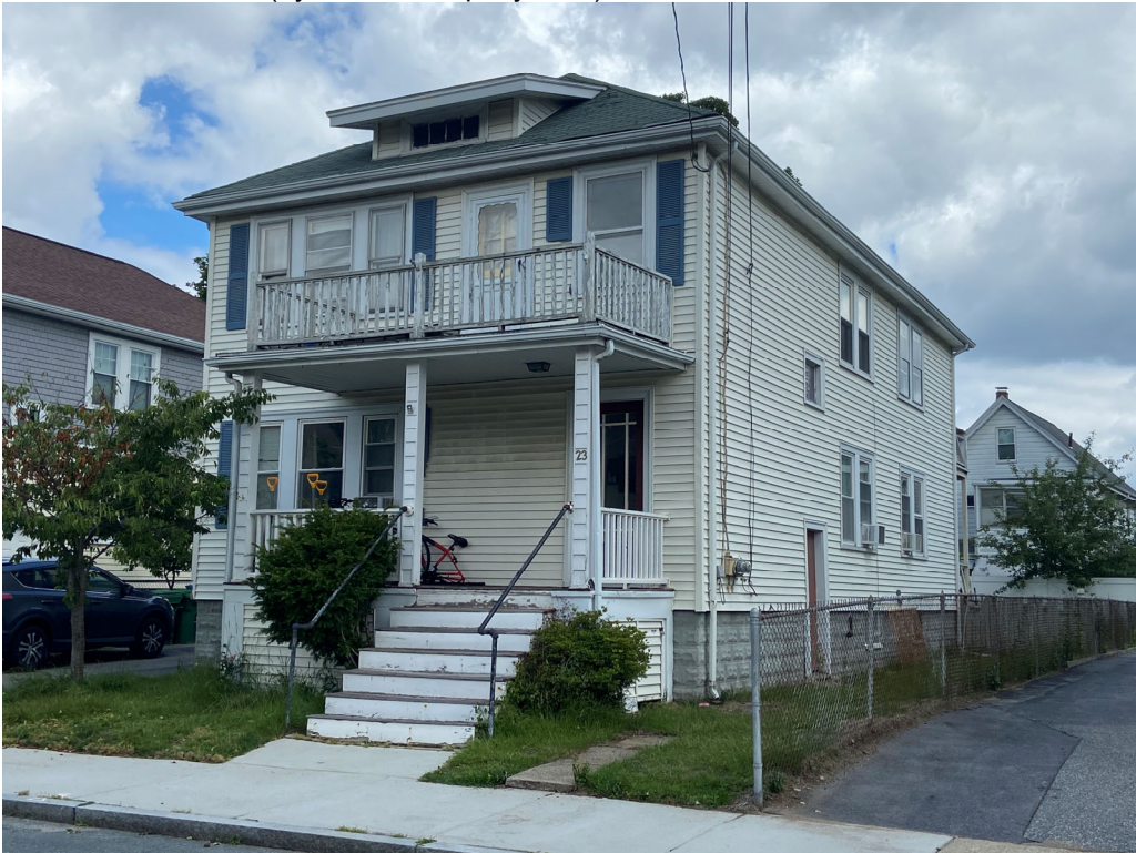
View from SE showing larger paired windows, stair light and cellar door.
