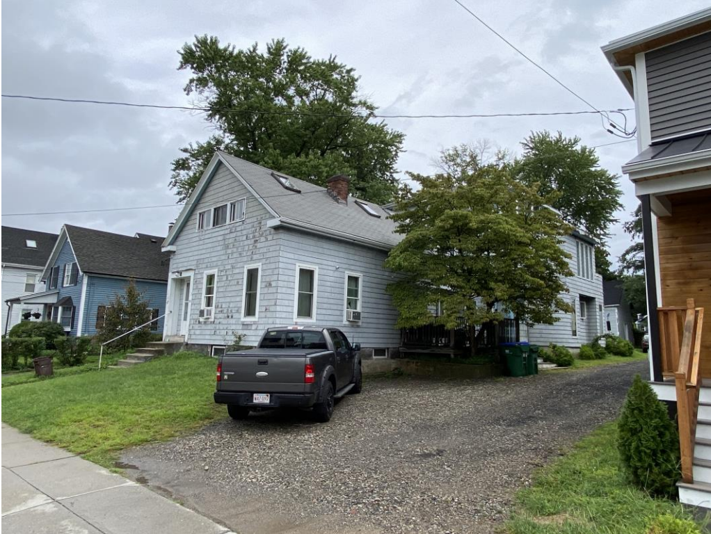
View from SW.
